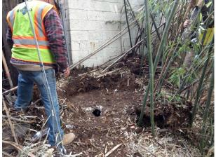
We then determined that the Parish House sewer line emptied into the manhole and verified it was clear and working. The Church line did not empty into the manhole which meant it connected to the Parish House sewer line somewhere between the Parish House and manhole. The City crew, using a divining rod system, located the Parish House sewer line, the Church sewer line and the location where the Church line connected to the Parish House line.
